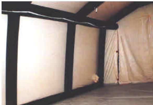
ample headroom on floor area
